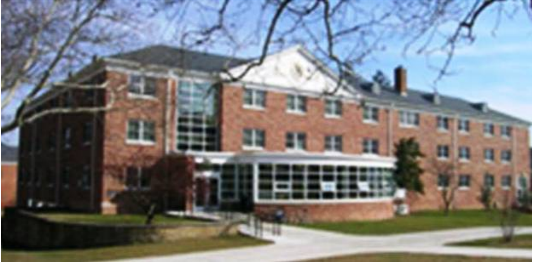
Lesher Hall – Built in 1957 Named East Hall until 1960
