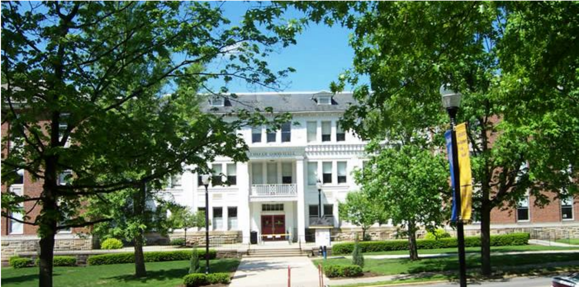
Good Hall (after expansion of Science Hall in 1967)
