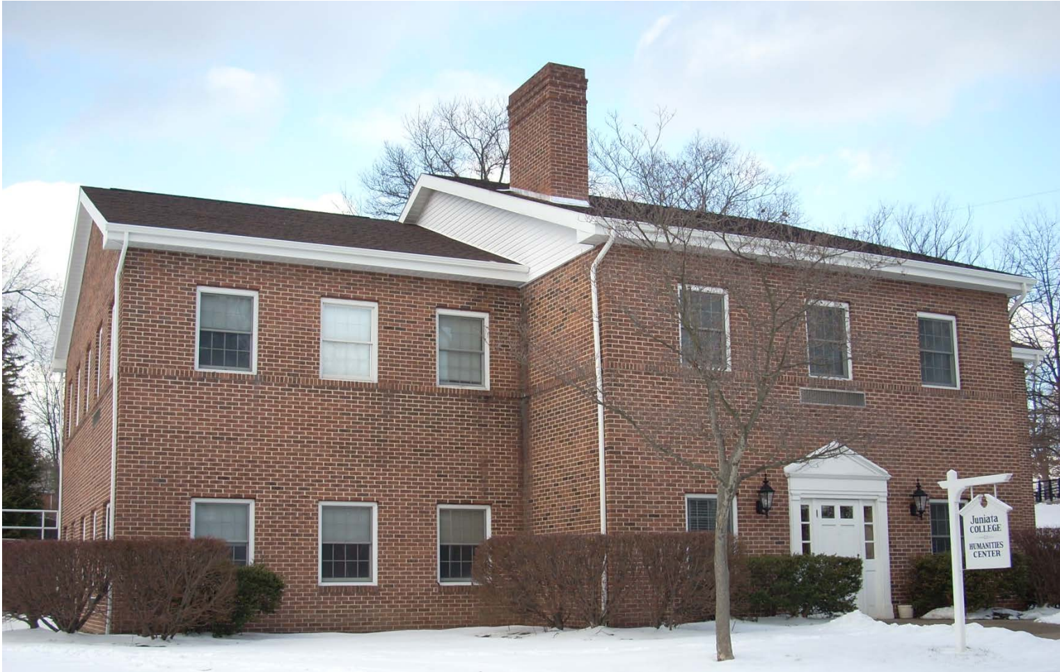
Humanities Building - Built in 1979
