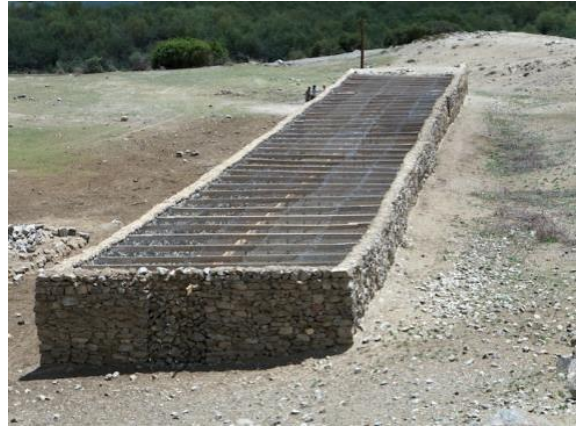
Figure 26. The same corral after being refurbished. Photo credit: Panthera.
