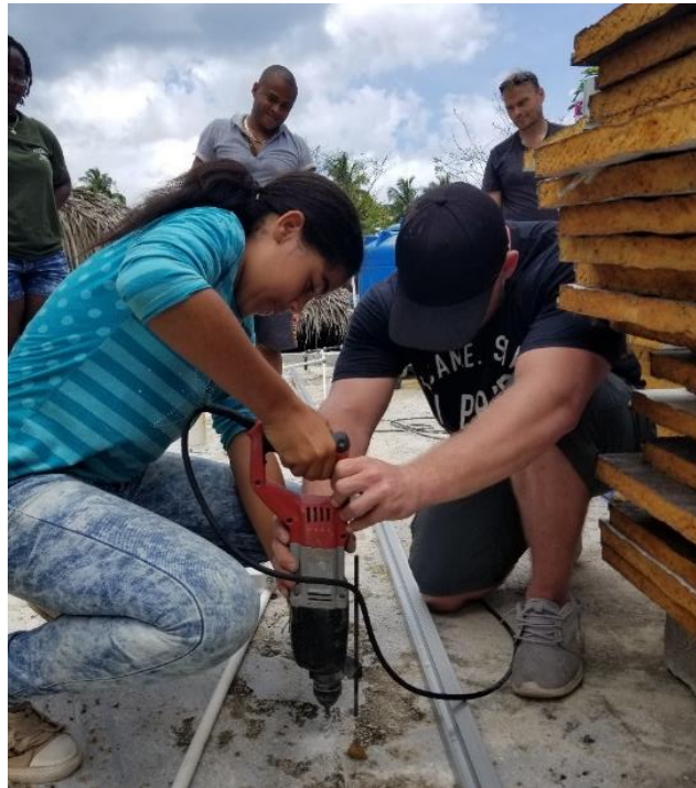
Figure 18. Lycoming Student Zach Staver works with a Las Terrenas International School student to install a solar system on the school's roof. Photo credit: Jeremy Ramsey.
